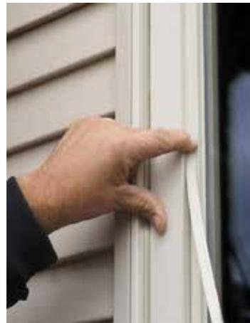
Caulk windows as well as caulking and weather-stripping doors. Keep the outside air out and the inside air in.
